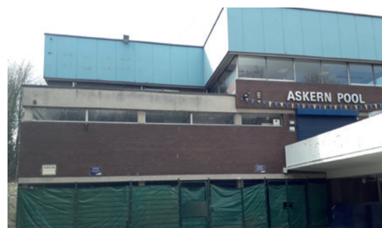
The Leisure Centre before refurbishment
